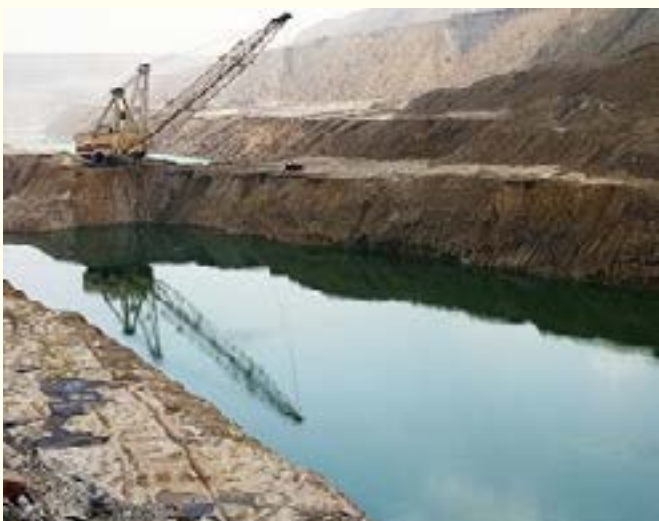
Fig.-11: Rise of water level in coal face
