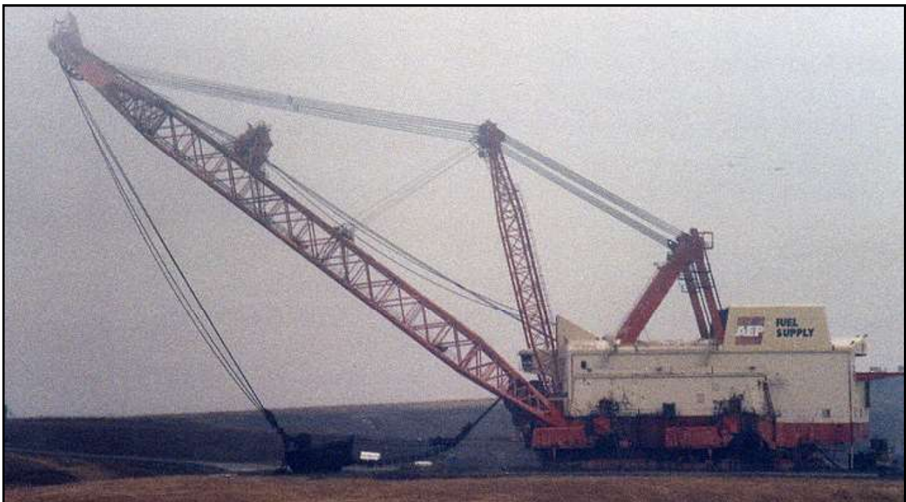
Fig. -1: “Big Muskie” prior to demolition in Ohio, February 1999
