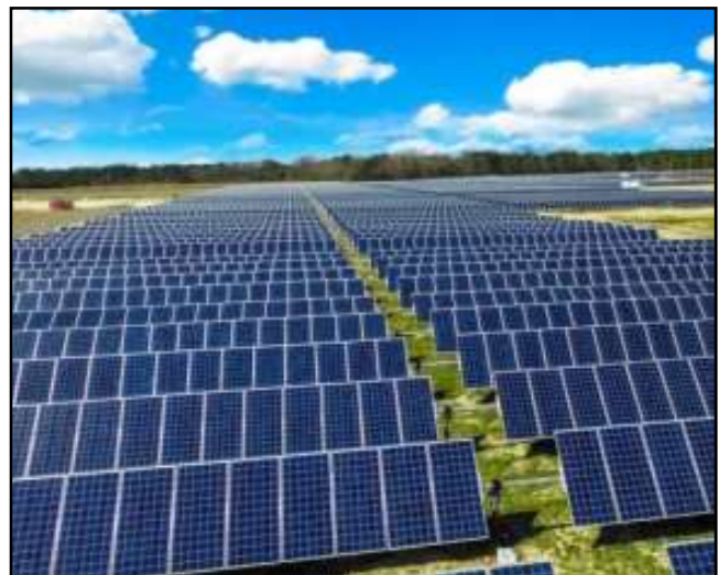
Fig-1: Laying of Solar panels in open ground
