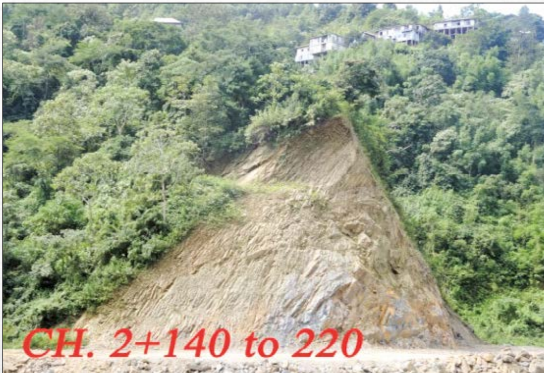
Plate-8: Final excavated road at Ch: +2150 m
