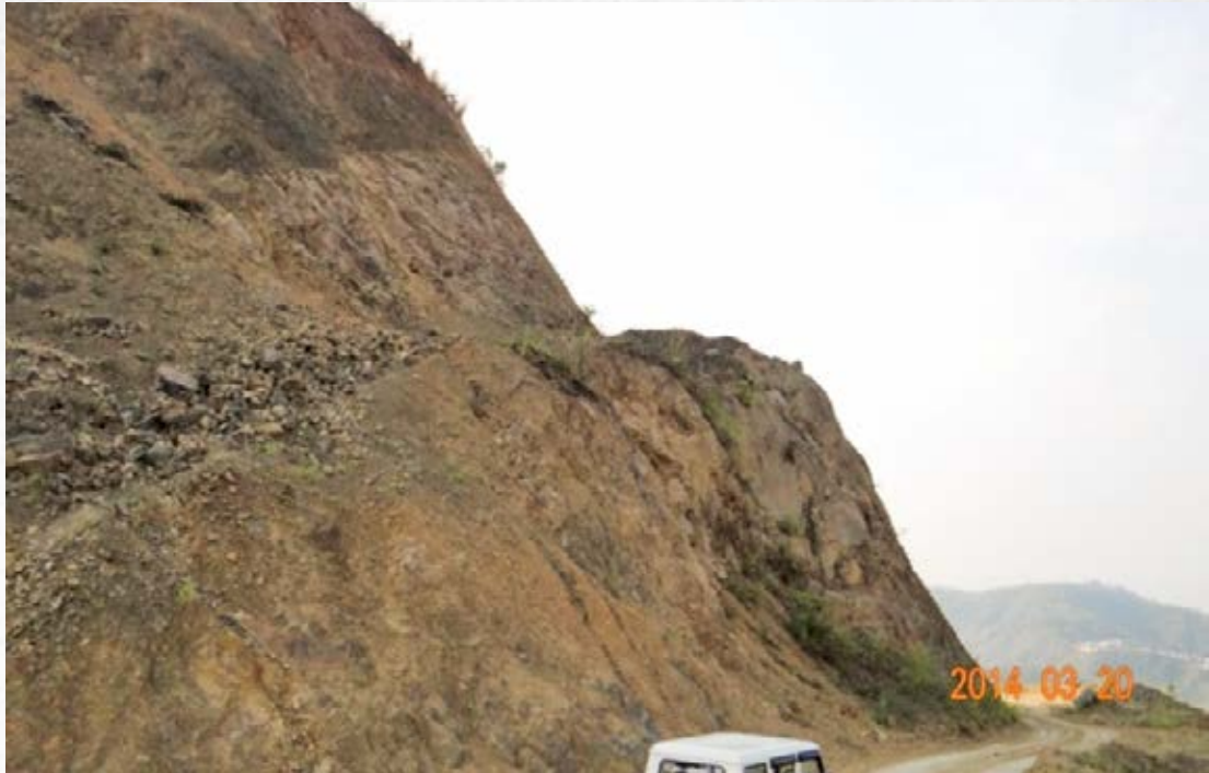
Plate-2: Closer view of the rock formation at Ch: +400 m
