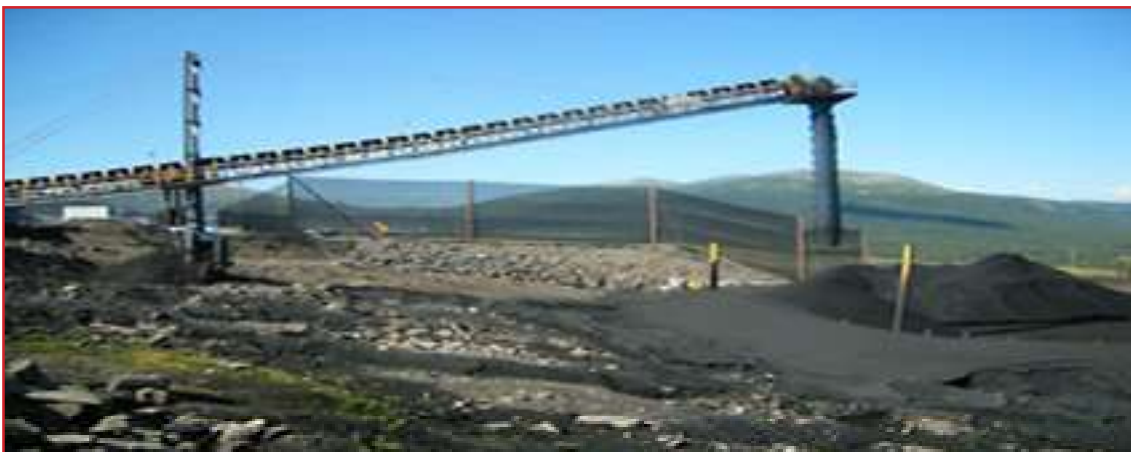
Figure 5: Wind Barrier around a coal dump
